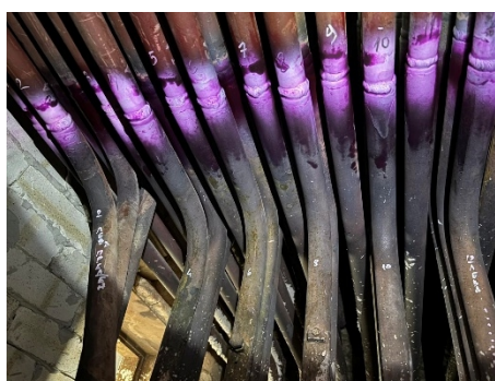
Figure 2. On-site welds (10CrMo9-10 and 12X1MF)
